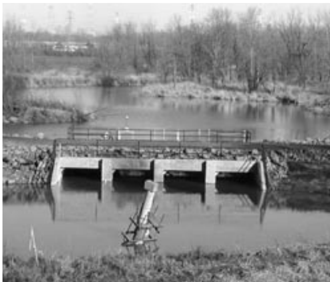
The new water-control structure at Smith and Bybee Lakes Wildlife Area reconnects the area with the Columbia River floodplain – and its past.
