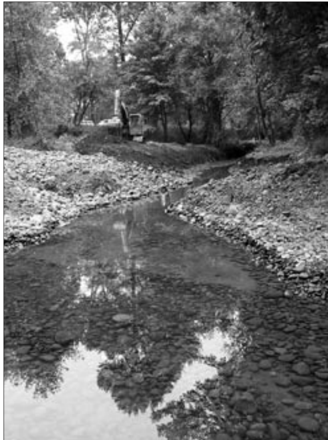
The new groundwater-fed lower channel provides year-round refuge for young salmon in the Clackamas River.
