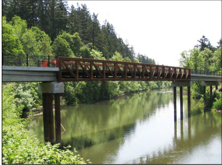
Image 9 Ki-a-Kuts Bridge over the Tualatin River
