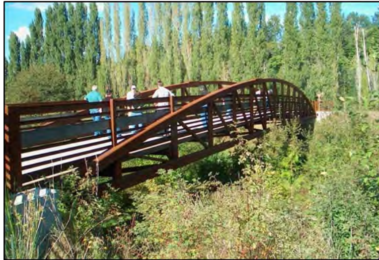
Image 4 Short bridge span
