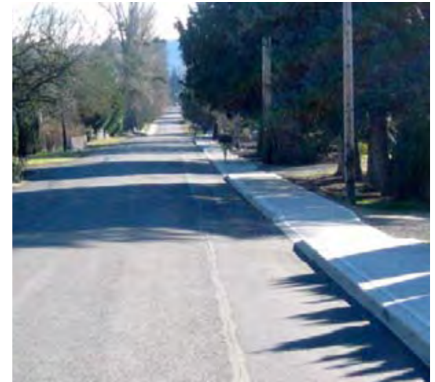
The recently completed sidewalk project on SW 173rd Avenue provides safe access for students at Aloha-Huber Park School.
