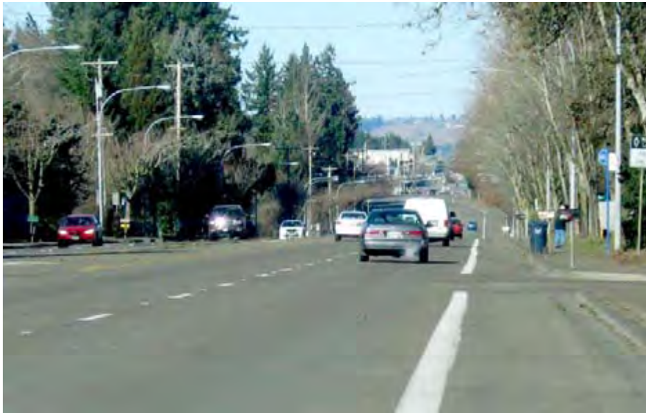
185th Avenue between Baseline Road and Johnson Street – a mile-long segment of five-lane roadway with bus stops and surrounding residential development – has no traffic signals or pedestrian crossings.
