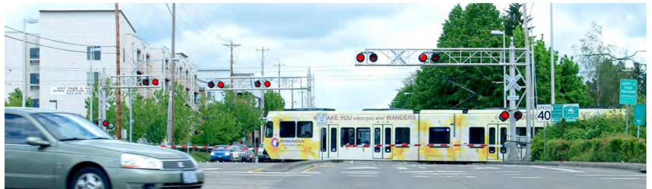
185th Avenue at Baseline Road
