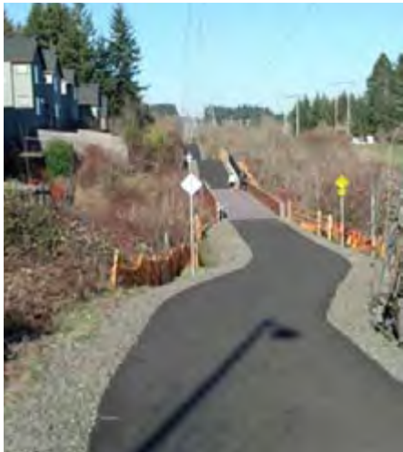
The Westside Trail is now complete from Blanton Street in Aloha to Barrows Road in the Progress Ridge area of Beaverton.
