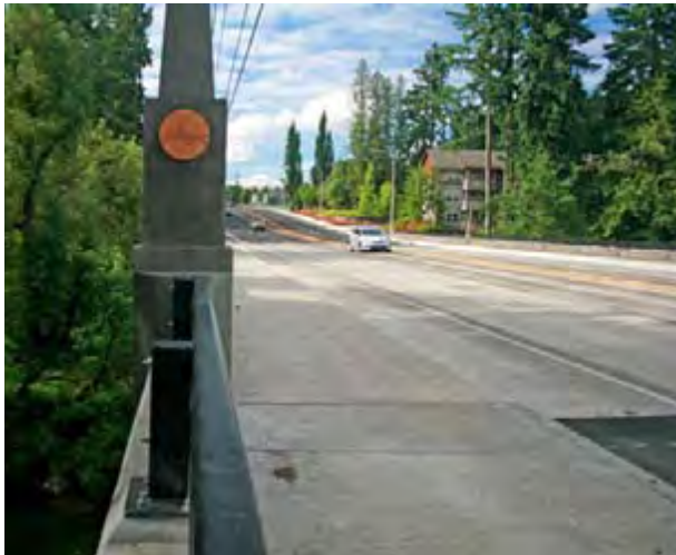
Bridge over Beaverton Creek, Cornelius Pass Road
