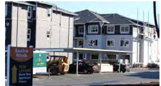
The Baseline Woods housing development will add over 450 housing units upon completion sometime in 2014.
