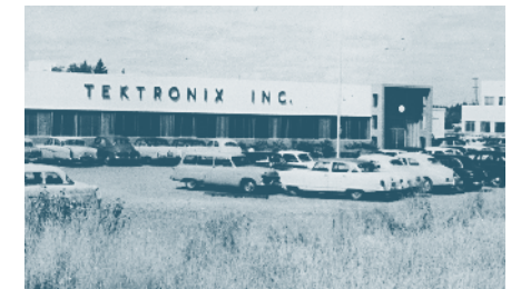
Opposite page: Ships and wharves along the waterfront in downtown Portland, circa 1900. This page, above: Tektronix, Inc., shown here in October 1954, was one of many new businesses seeking good sites that moved into the Tualatin Valley in the 1950s, shifting the economic base of an area that had once been primarily agricultural land.
