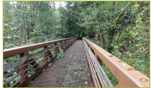
Existing bridge over Mount Scott Creek in Mount Talbert
