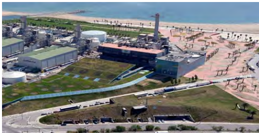
Barcelona, Spain waste to energy plant
