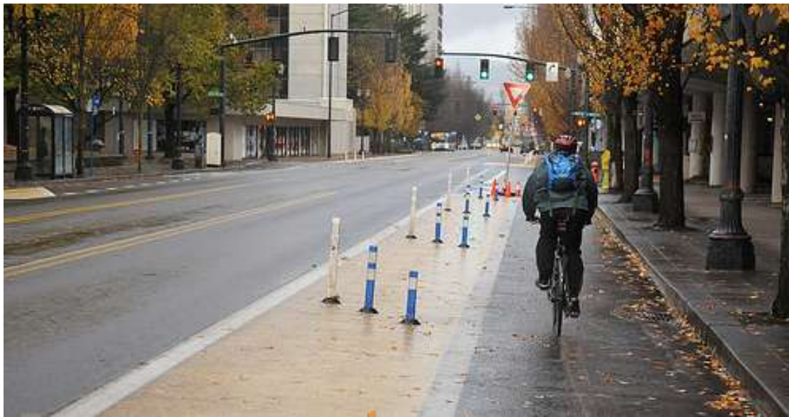
Multnomah Boulevard cycletrack in Portland provides a safe direct route making bicycle travel easy. Photo: BikePortland.org
