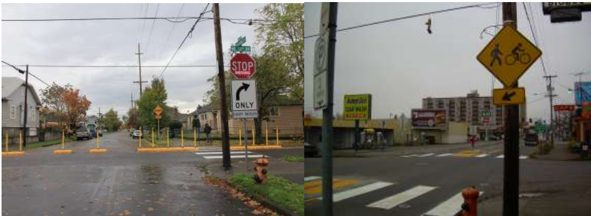
The photo on the left shows a bicycle crossing treatment on NE 33rd Avenue in Portland. The crossing treatment also diverts traffic from the bicycle boulevard on Going Street. The photo on the right shows a sign alerting drivers of a pedestrian and bicycle crossing along the Spokane Neighborhood Greenway. Photos: Portland, Greg Raismen
