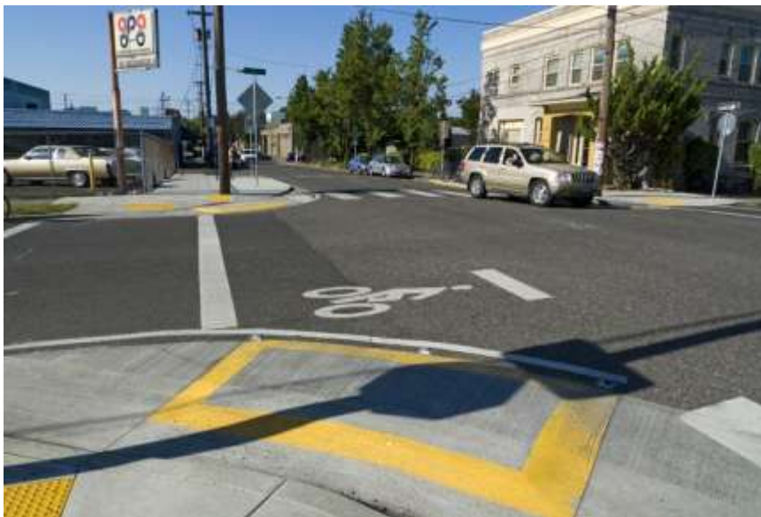
Example of a truck apron, extending the curb making it easier for pedestrians to cross the street, but maintains the turning radius for large trucks which can mount curb. Photo: Michael McKisson.
