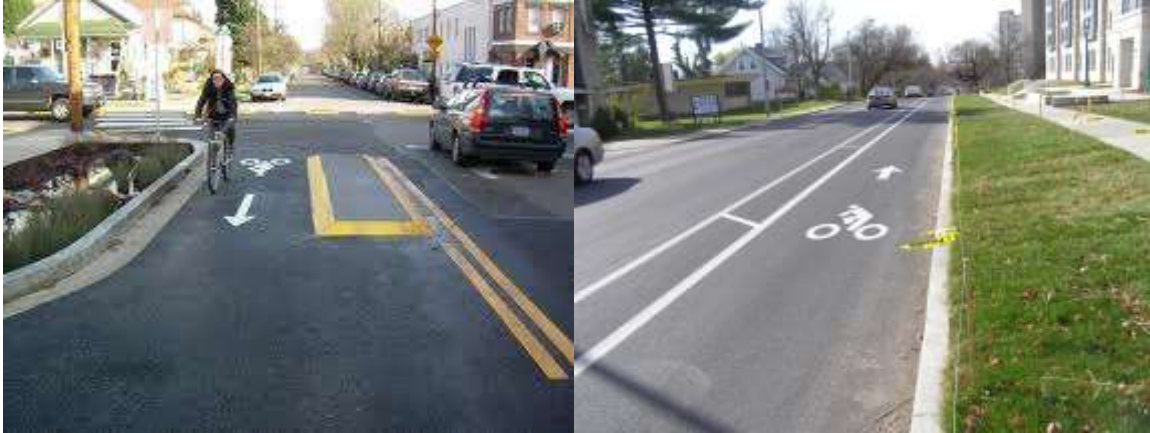
The photo on the left shows a traffic calming treatment at the entrance to a bicycle boulevard. A bioswale narrows the street. Two way bicycle traffic is allowed while autos may only exit. The photo on the right shows a buffered bicycle lane on a lower traffic street in Bloomington, Indiana. Photos: Portland, City of Bloomington
