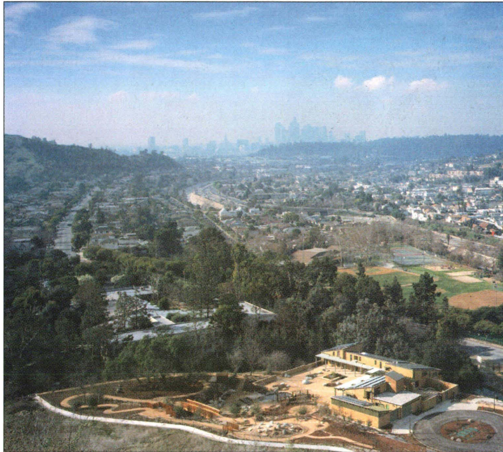
Inverters from Arlington, Wash.-based Outback Power Systems turn solar rays into power at the Los Angeles Audubon Society.
