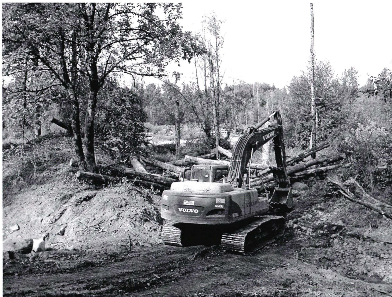
Log jam construction
