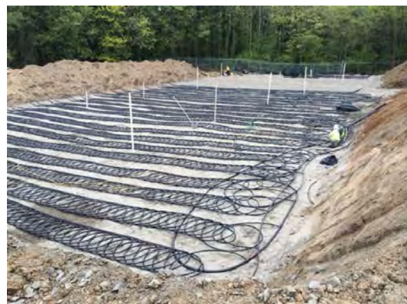
Subterranean geothermal system installation in progress at the Oregon Zoo.
