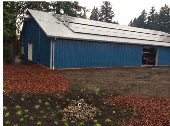
The solar array on the Glendoveer golf cart barn will produce 23,737 kWh of electricity per year.
