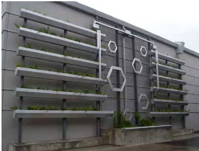
Portland Expo Center green wall. Photo courtesy of GreenWorks
