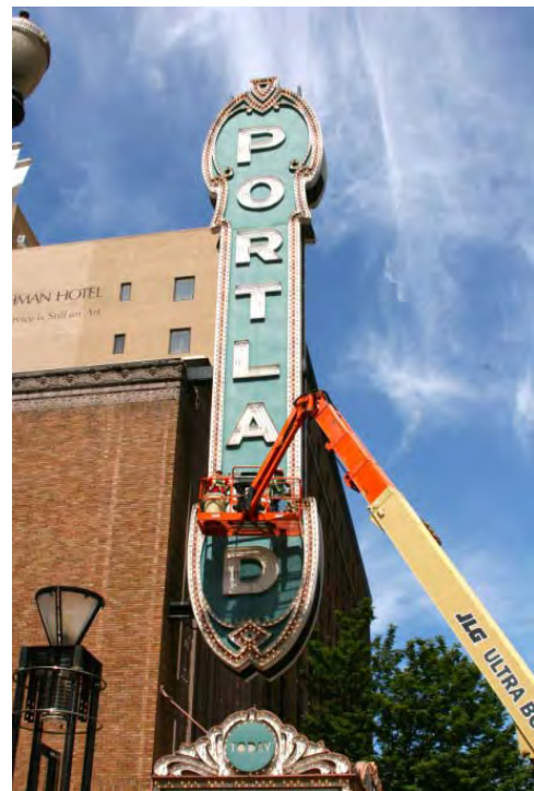
Energy hogging 11-watt bulbs were swapped out for super efficient 2-watt LED's on the Portland marquee. Photo by December Carson.
