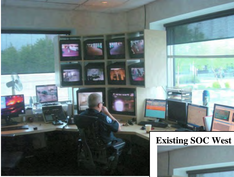
Existing SOC SW Corner
