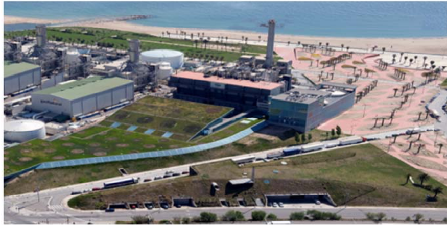
Barcelona, Spain waste to energy plant
