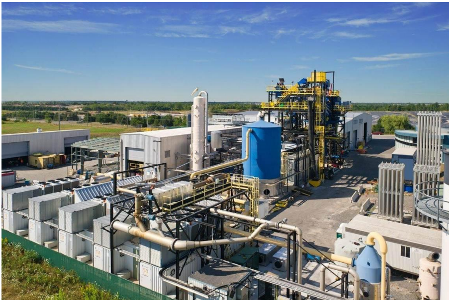
Computer Drawing of the Proposed Plasco Energy Plasma Arc Gasification Facility in Ottawa, Ontario
