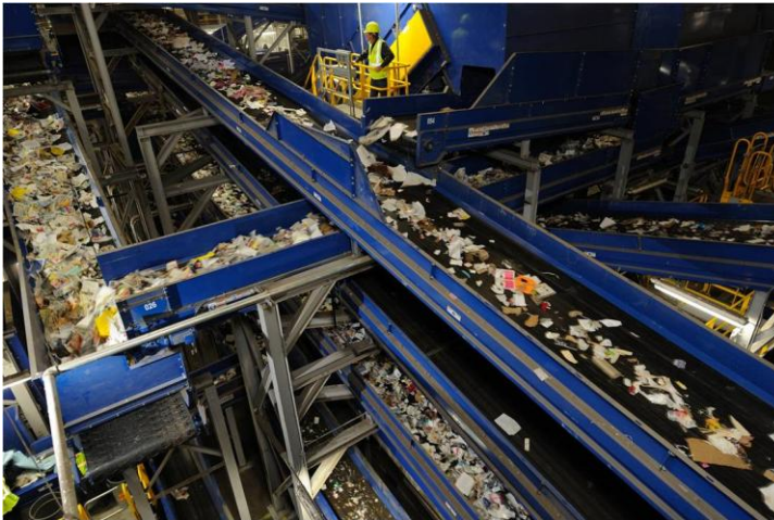
Republic Services' Newby Island materials recovery facility in Milpitas CA
