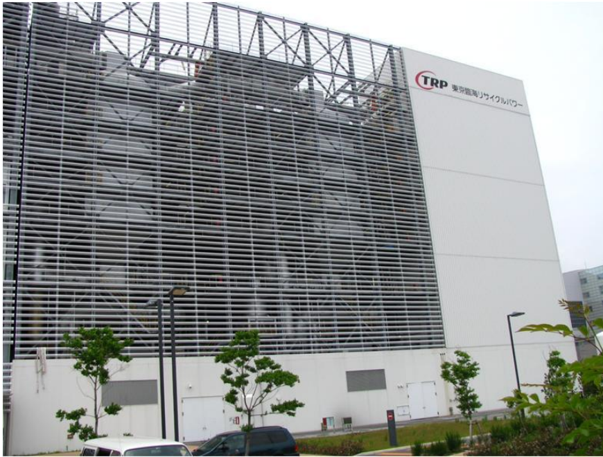
*HDR Photo of TRP Gasification Plant in Tokyo, Japan
