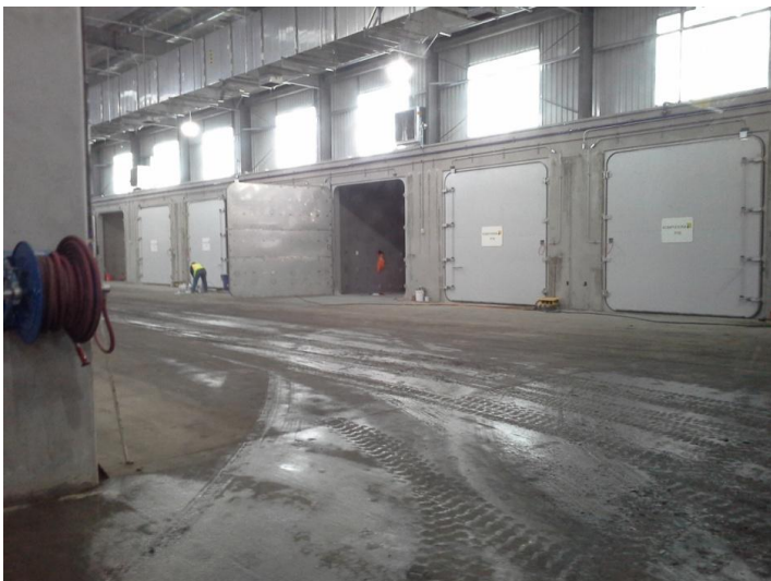
Example of Bunker type - Dry Fermentation Process Photo inside of San Jose ZWED facility
