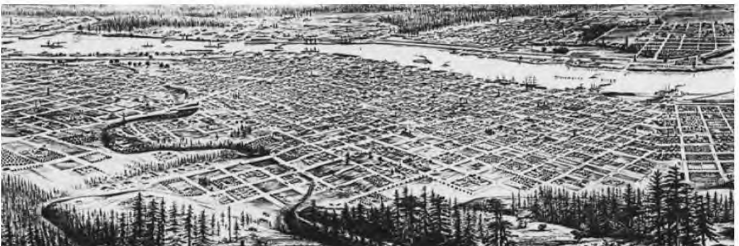
Early platting from the 19th Century looking east across downtown
