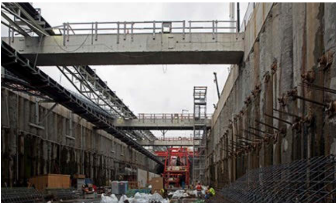
Cut-and-cover construction for the downtown tunnel in Seattle (1980s)
