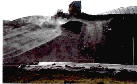
Tipper At Working Face
