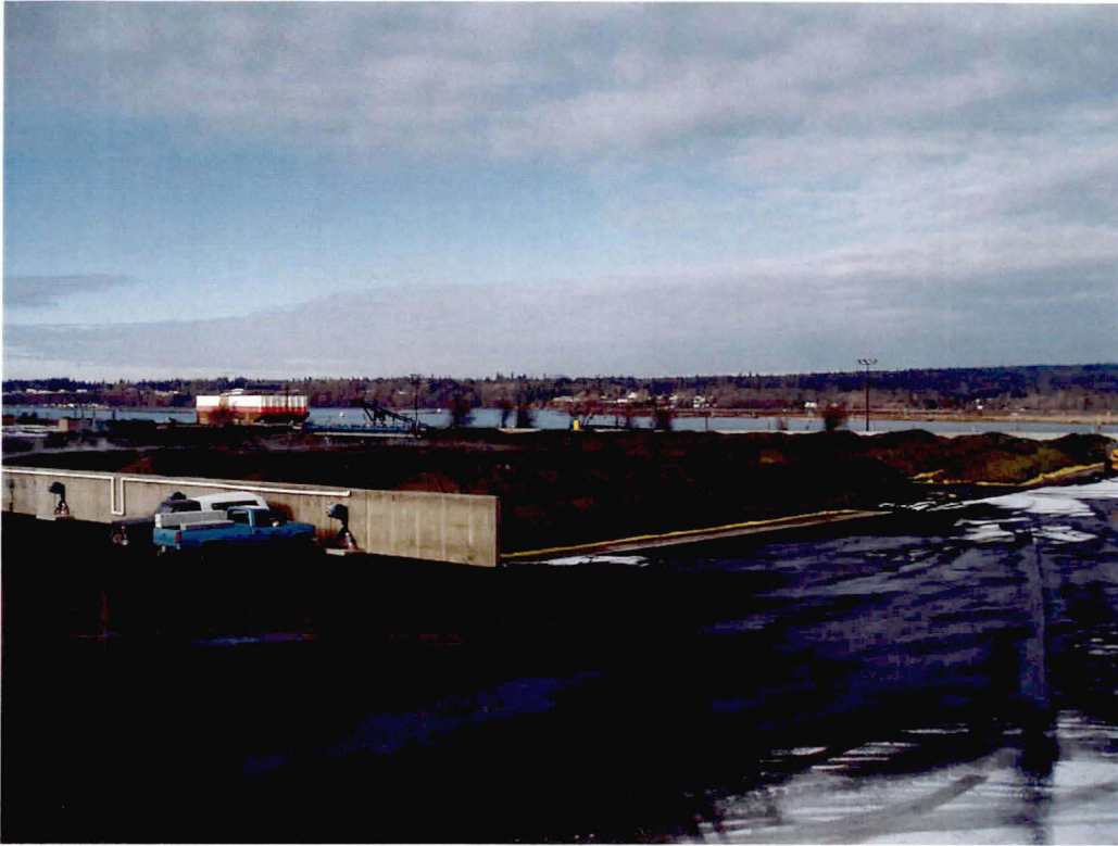
Cedar Grove's Everett Facility
