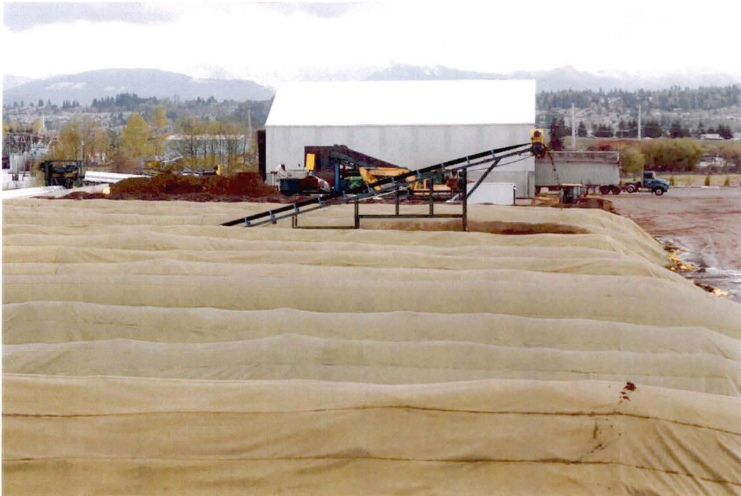
Cedar Grove's Maple Valley Facility
