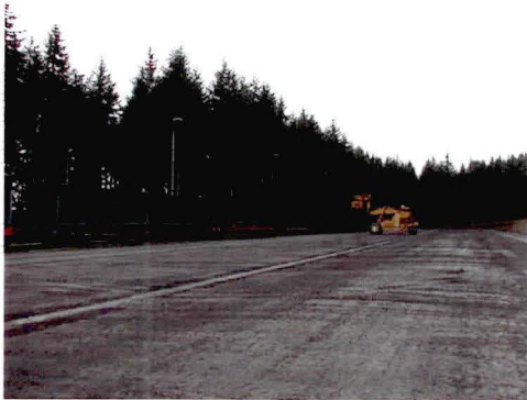
Rail Siding At Landfill
