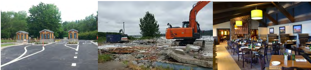
The new Blue Lake entry, removal of the Gleason Boat Ramp portage building, the Ringside after renovations
