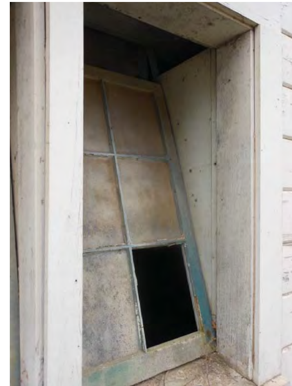
Repair & Replace Windows
