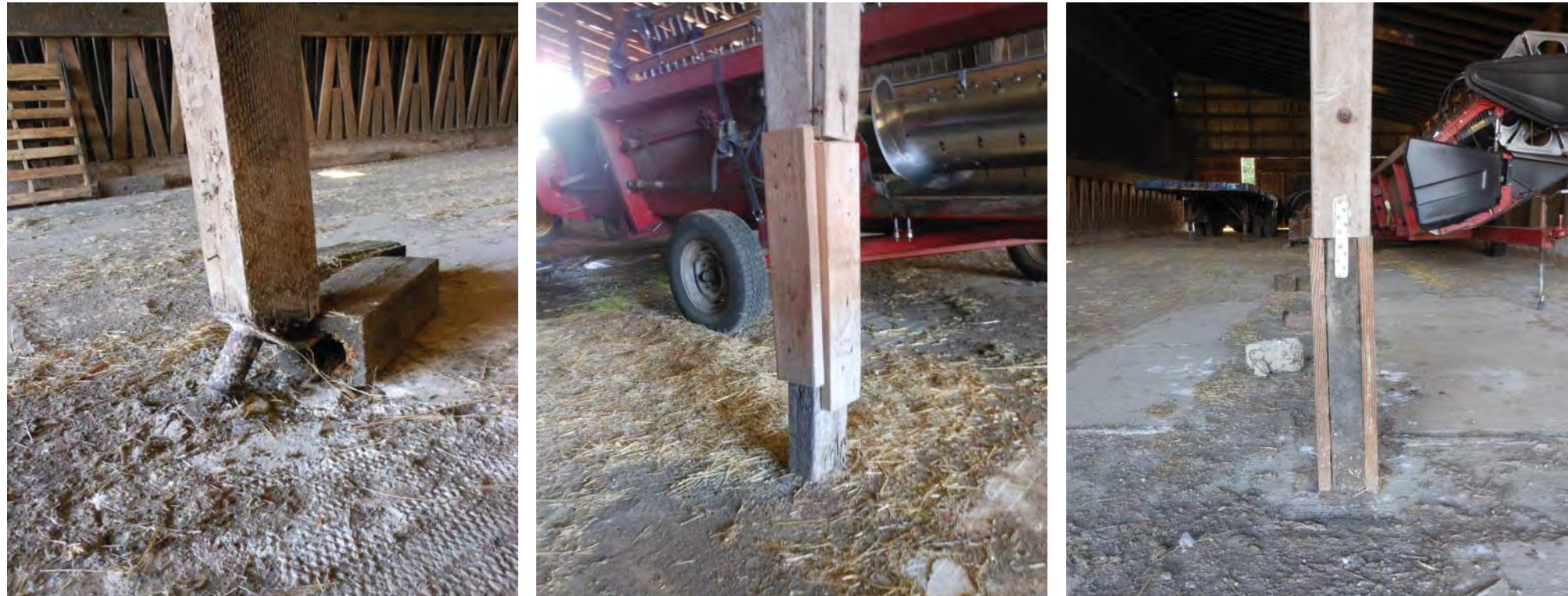
Column Bases at Accessory Barn #1. These columns could be a safety hazard and should be suitably reinforced or replaced.
