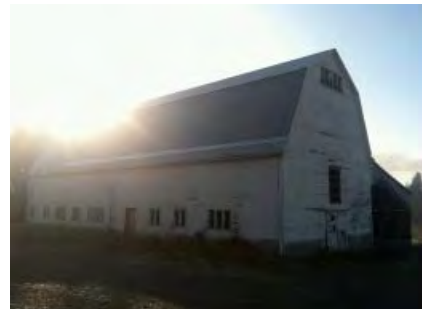
North side of barn
