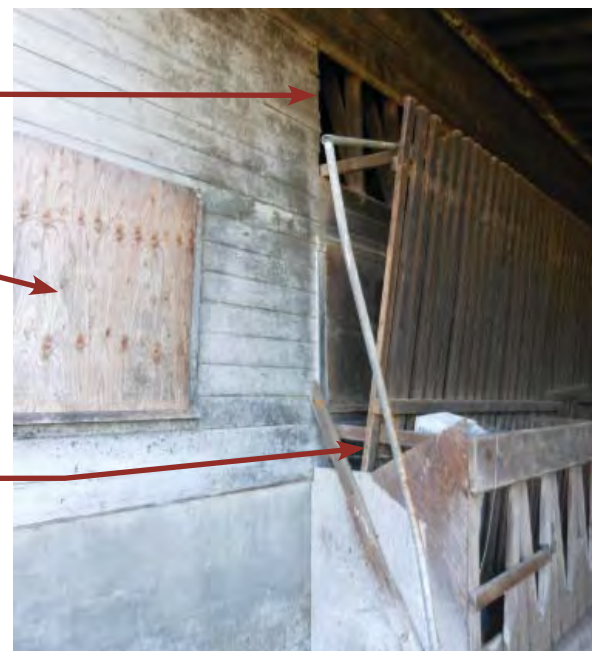
SIDING REMOVED AT SOUTH SIDE OF MAIN BARN
