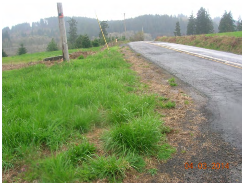
West access looking west
