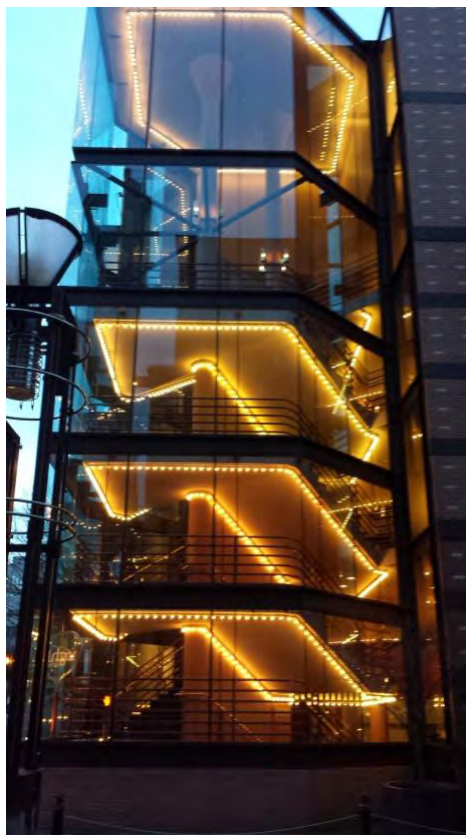
Portland'5 Centers for the Arts replaced 4,000 light bulbs at Antoinette Hatfield Hall saving 148,000 kilowatts of electricity per year.
