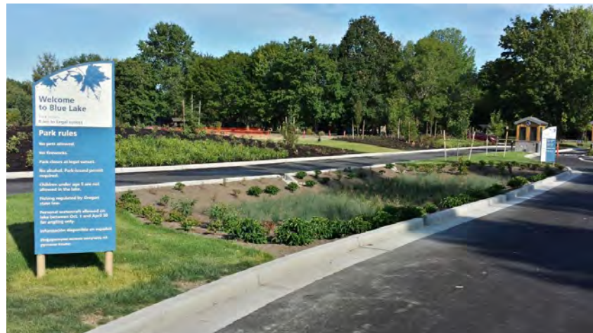
A new rain garden at the entrance of Blue Lake regional park treats stormwater runoff from 30,000 square feet of impervious area, protecting groundwater.
