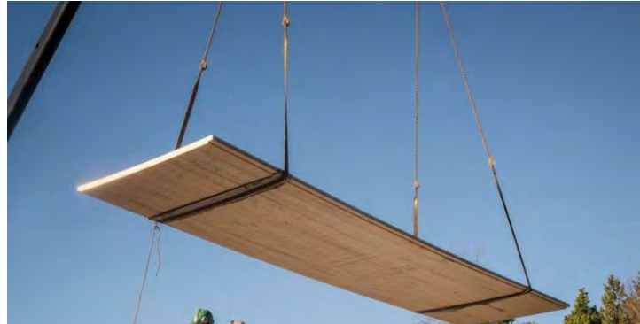
Cross laminated timber is lifted onto the roof of a building under construction for Elephant Lands at the Oregon Zoo.
