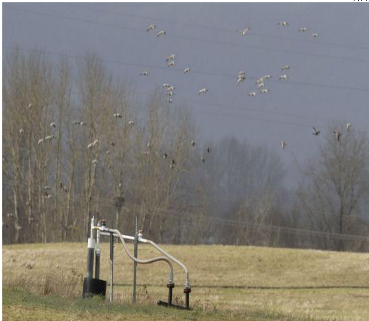
Landfill today with methane gas pipes
