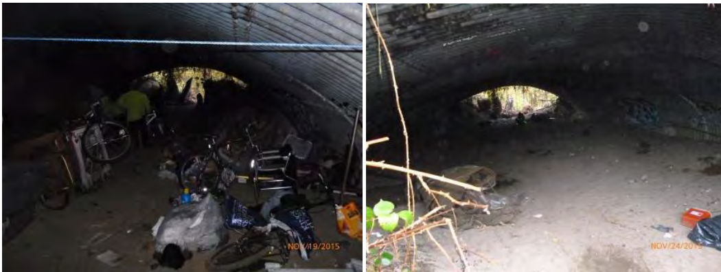
Before and after: Smith & Bybee Lake culvert cleanup
