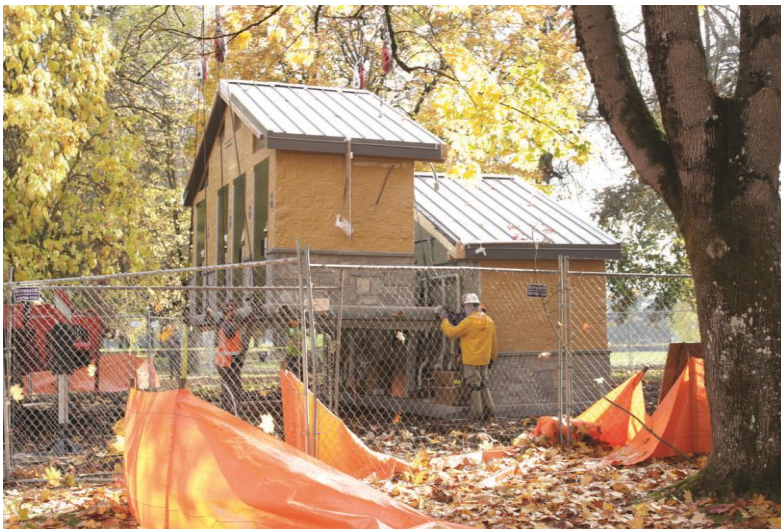
Prefabricated restrooms being craned in at Blue Lake Regional Park
