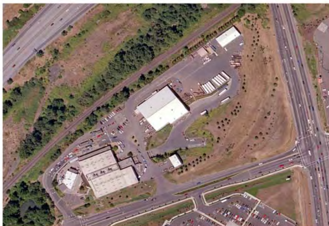
Metro South Transfer Station
