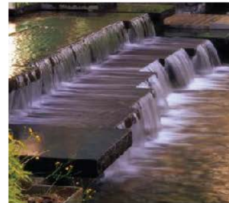
STONE WEIR SPILLWAY – INSPIRATION
