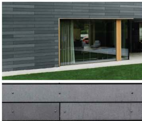
GFRC PLANK CLADDING WITH EXPOSED FASTENERS
