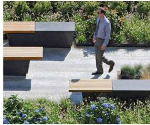
FIXED CUSTOM BENCHES – CIP CONCRETE AND WOOD
