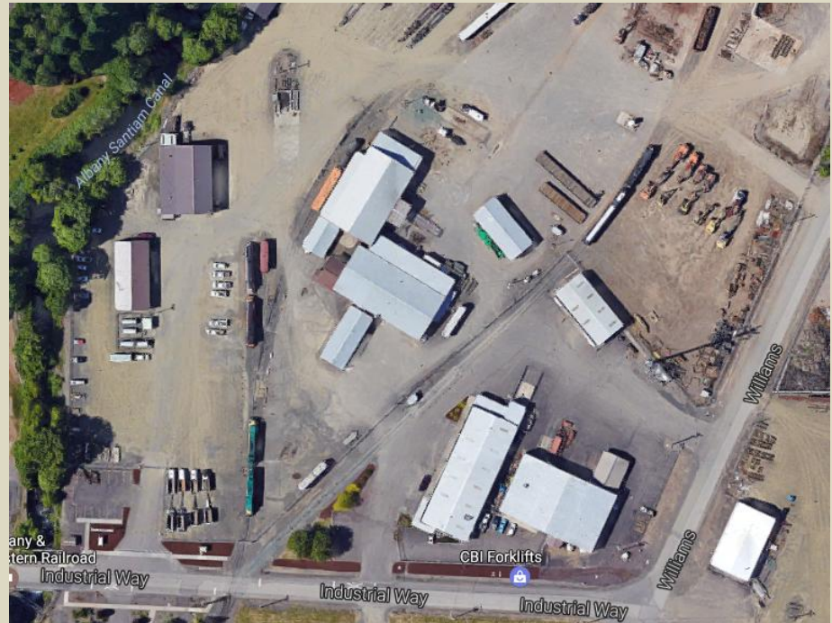
AERC Reload Facility in Lebanon
