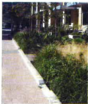
GREEN: stormwater planters filter runoff and create a pleasant transition from public to private space. Ecoroofs help to filter stormwater runoff and should be incorporated in building design whenever possible
