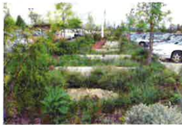
Parking Lot Rain Garden (Natural detention and filtration of parking lot rainwater)
