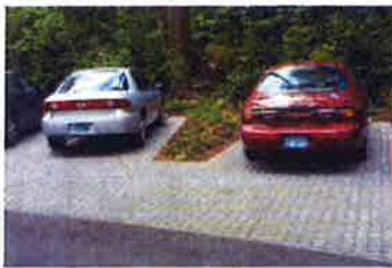
Pervious Paving (Allows rainwater to percolate into soil)
