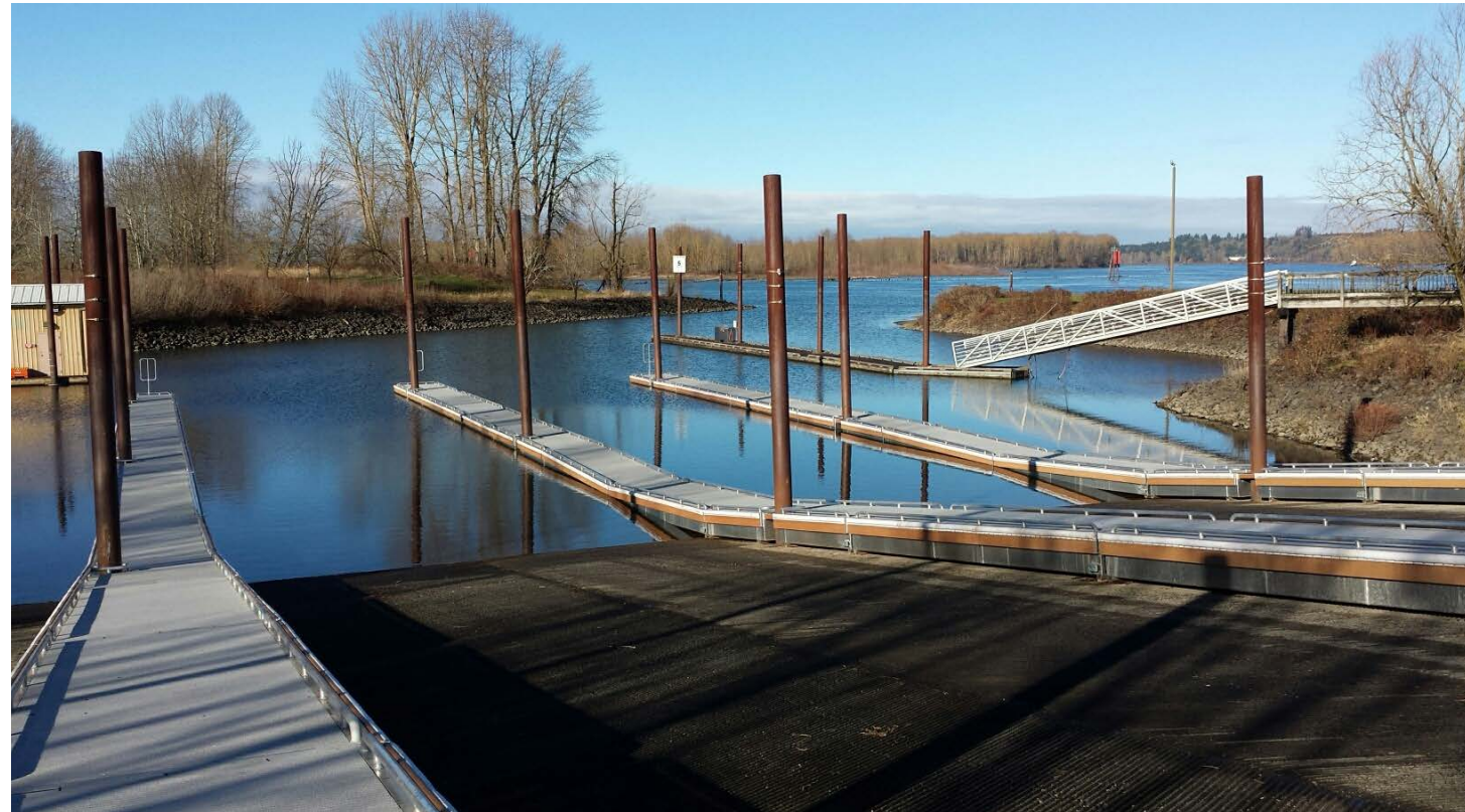
Chinook Landing boat dock replacement
