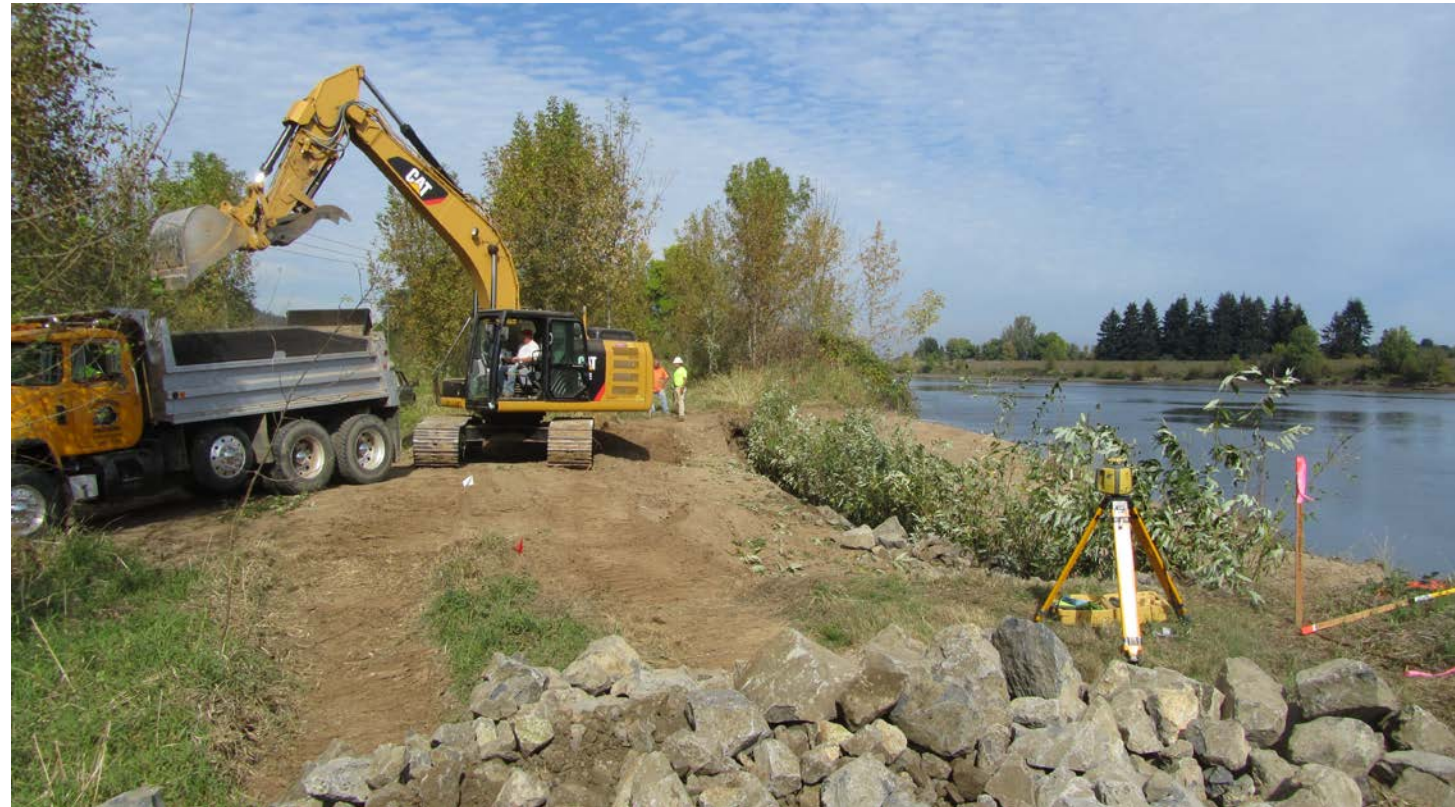
Multnomah Channel spillway construction
