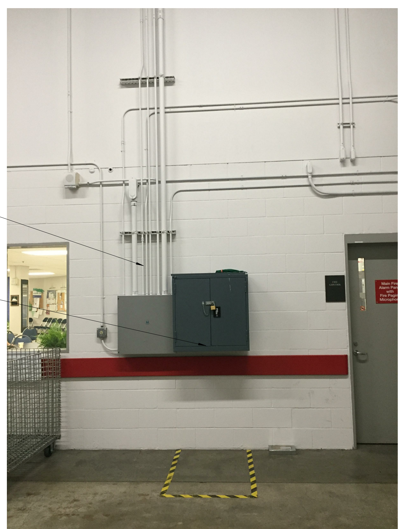
CORRIDOR ELEVATION IMAGE - FOR REFERENCE
