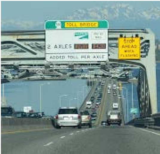
Bridge reconstruction/ replacement
