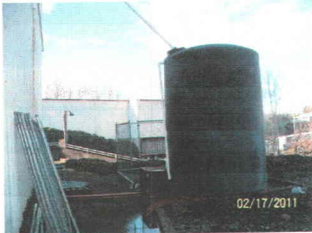
Figure 2 5000 gallon rain water storage tank behind the truck wash
