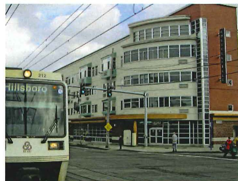
Photo: Thomas Harris Architects: MWA Architects Developer: HomeForward
