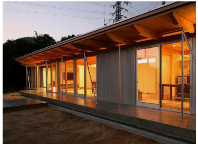
This 1,100 square foot modular home by Anderson Anderson Architecture was constructed in Japan with a budget of $154,000. This works out to about $140/SF. Source: Anderson Architecture
