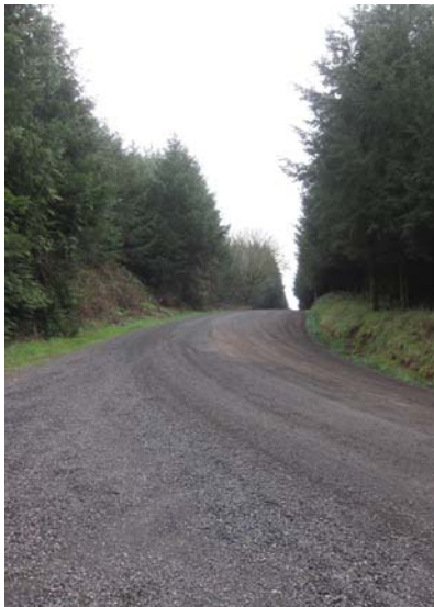
Southwest Dixon Mill Road, looking east from existing gated access point
