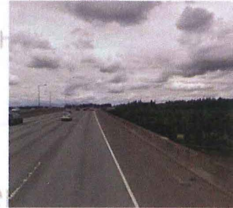
Glenn L. Jackson Memorial Bridge Interstate 205 - Columbia River
