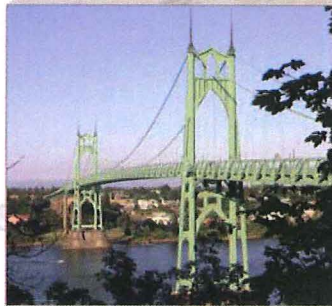
St Johns Bridge US 30 Bypass - Willamette River West Slope
