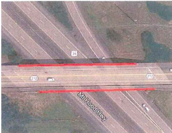
Bridge #13492, Hwy 174 over Hwy 26, 505' Protective Fence
