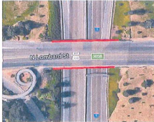
Bridge #08996, N Lombard St over I-5, 286' Protective Fence
