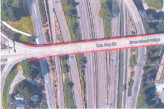
Bridge #05054, US26 Ross Island Bridge over I-5, 993' Protective Fence
