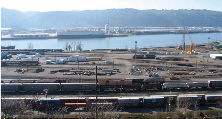
Class 1 railroads like the Union Pacific rail yard in North Portland are experiencing capacity constraints.
