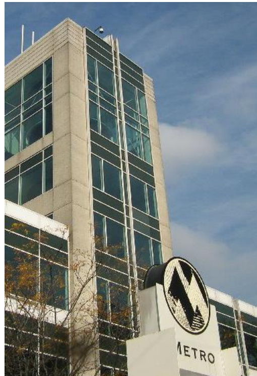
Manage Metro Regional Center campus
