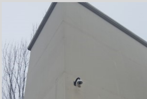
Source: Metro Auditor’s Office photo of surveillance camera at Metro Regional Center.
