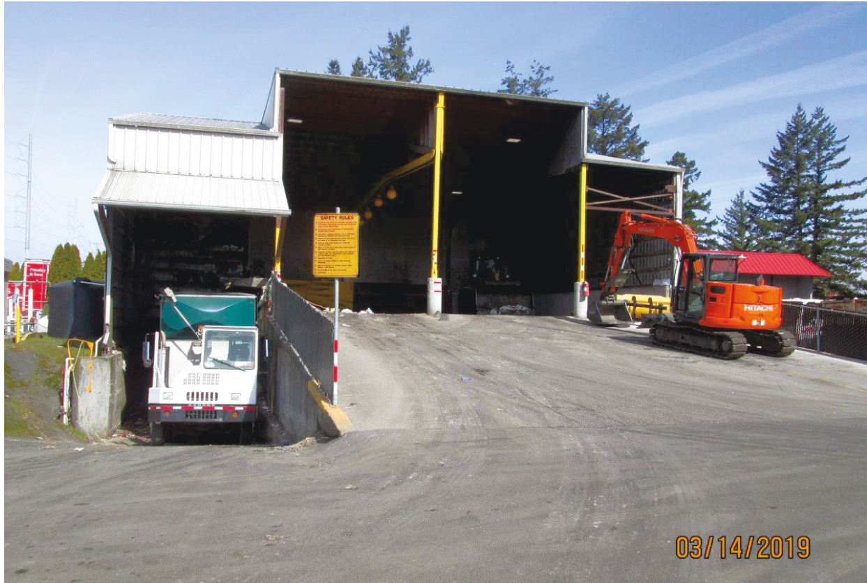
Photo 2: GSS Transfer located at 2131 NW Birdsdale Ave. in Gresham
