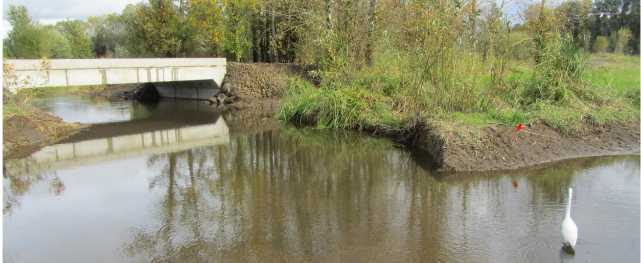
This photo shows the new bridge, constructed in the central access road in 2014. The stream connecting the two wetland basins, which was realigned in 2008, can be seen flowing below the new bridge. Prior to 2014, the stream flowed through a triad of 36" culverts. Prior to 2001, the road had no gaps, and the two wetland basins were completely isolated from each other.
