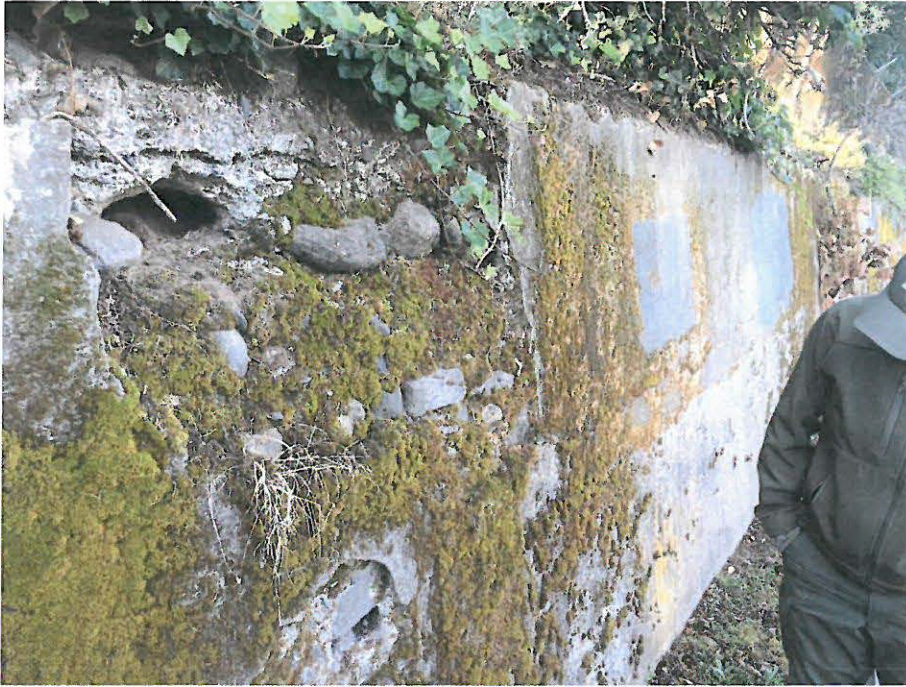
Photo 3 – Close-up of deteriorated portion
