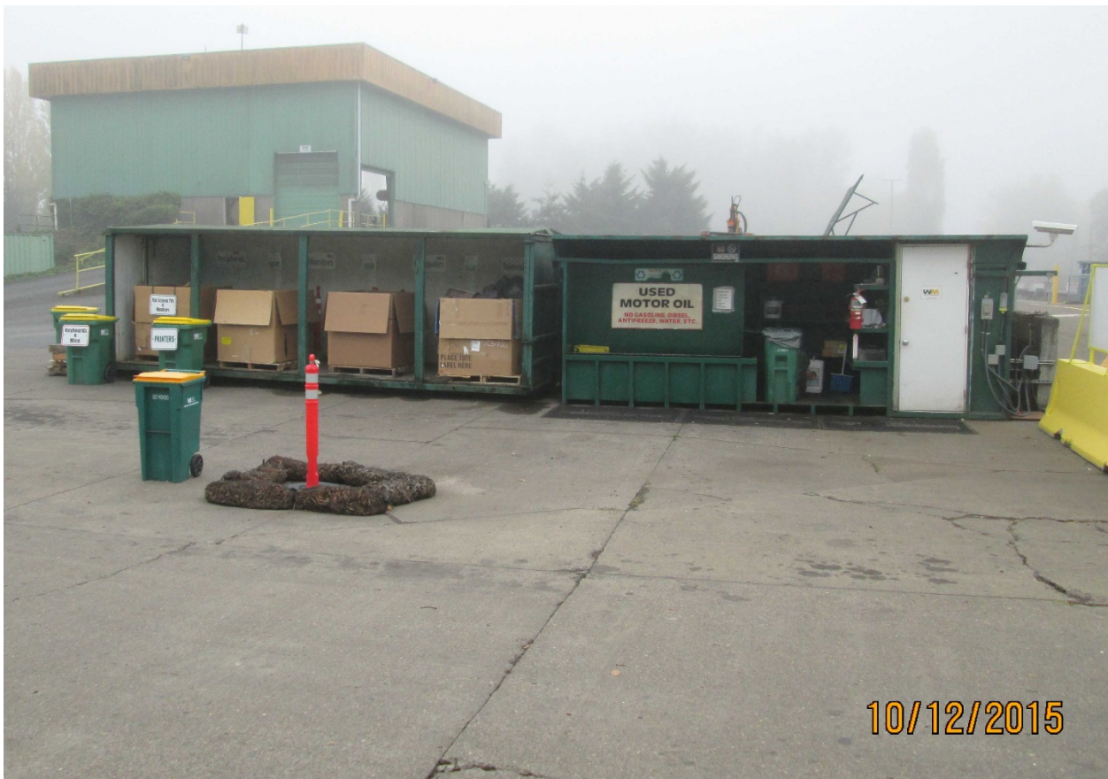
Photo 5: Forest Grove Transfer Station located at 1525 B St. in Forest Grove
