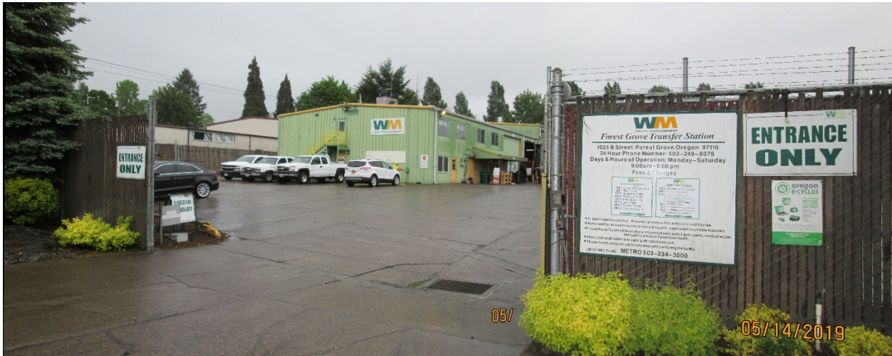
Photo 4: Forest Grove Transfer Station located at 1525 B St. in Forest Grove
