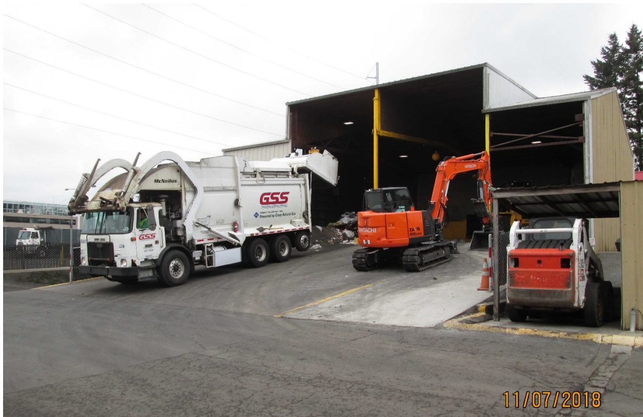
Photo 5: Gresham Sanitary Services located at 2131 NW Birdsdale Ave. in Gresham
