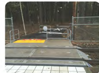
rail road crossing
