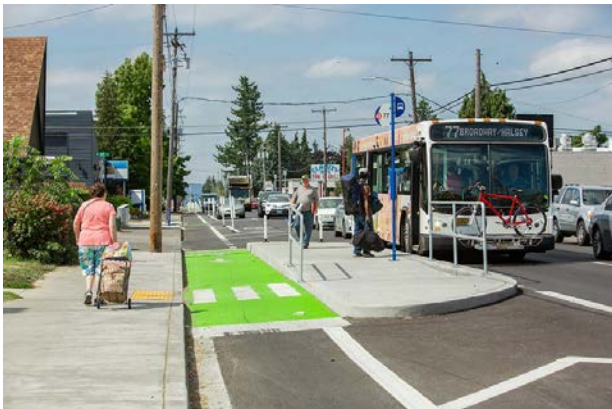
Bike, Pedestrian and ADA treatments on NE Halsey Photo courtesy of Metro
