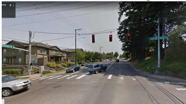
NW Division Complete Street Project western limits NW Division Street at Birdsale Ave looking east
