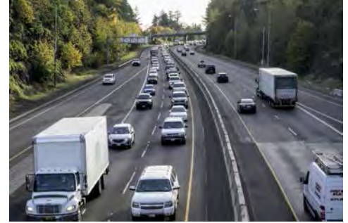
I-205 Project Corridor
