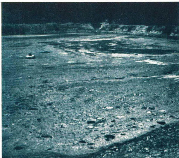
Lagoon shown is at Top-O-Topanga, California. A heavy growth of algae and floating sewage have made aeration impossible. Odors coming from this lagoon were very offensive.
