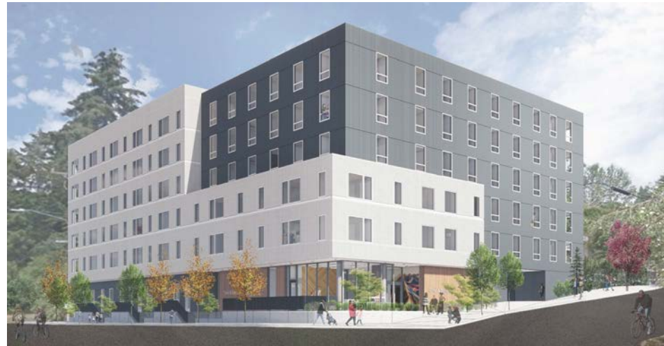
Viewfinder, 81 units in Tigard Community Development Partners | Opening Fall 2021
