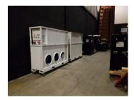
New chilled water air handlers have arrived at the Keller-a process that took approximately 18 months. These will provide cooling for the stage-that has never had its own cooling system. In the past, the stage could do fine from cooling in the audience but heavy tech Broadway shows are pumping more and more heat on the stage, making it hard to keep cool in hot weather. In 2019 outside units had to be rented in order to maintain stage temperatures required by Actors Equity.
