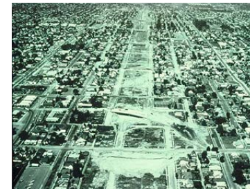
15 Photo: Destruction of Albina for Interstate 5
